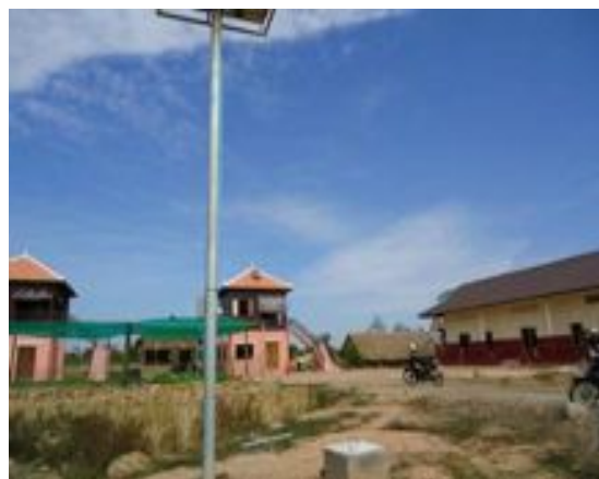
View of building in residential center
